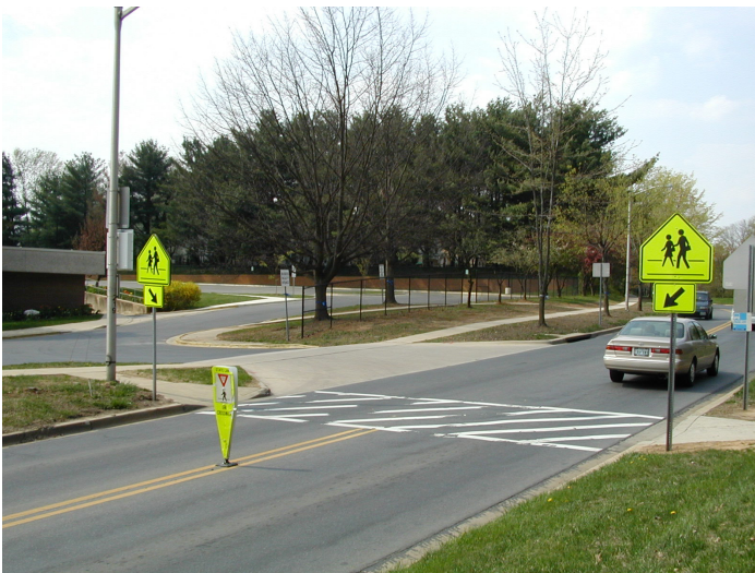
Pedestrian crossing signage
