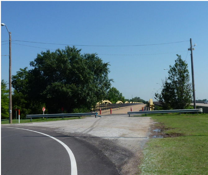
When the newer 96th Street bridge was constructed, Jenks maintained the old one, pictured here at left, for bicyclist and pedestrian travel.
